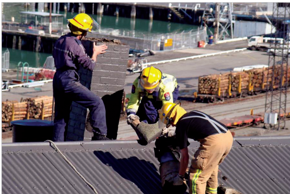
PHOTO 4. Lyttelton Fire Brigade dismantling a dangerous chimney.
